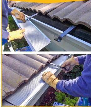
VILA TILE ROOF
